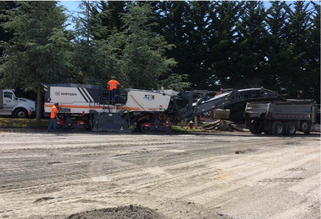
TCE Parking Lot Repave
